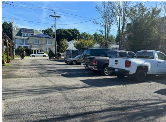
View of the third ingress and egress point along Bloomfield Avenue. This access drive and parking area is on the eastern side of the large wood trellis that divides the parking lot into two areas. Like the other parking areas, the parking spaces are undefined.
