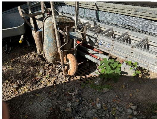
View of the southwestern corner of the property (above left), which is the lowest point from the highest along the northeastern corner. It appears that water has eroded a channel into the gravel and soil over time. There is only one storm drain on the property (above right) which is partially obscured by junk and equipment. Based on our discussions with the property owner, this area floods periodically due to insufficient drainage.
