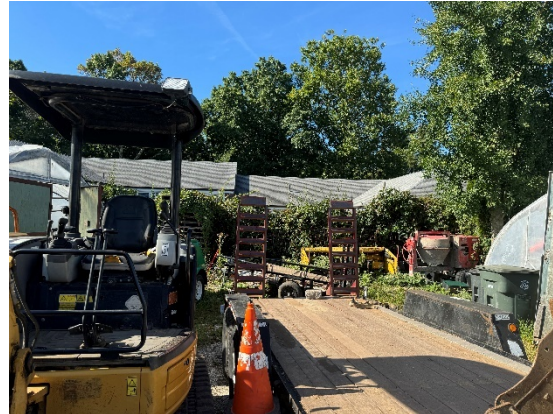
View towards the southerly property line showing the area between the three greenhouses to the rear.
