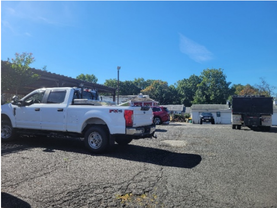
View of the parking lot looking inwards from Bloomfield Avenue, with the principal building to the right (not seen in the image) and the standalone plant display to the left. The parking lot is undefined as there is no differentiation between the access drive and the parking spaces. Lack of a loading space as seen by the truck parked to the right, proximate to the vehicles parked in the undefined parking spaces.
