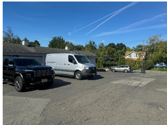
View of the ingress and egress along Park Avenue and the parking lot.
